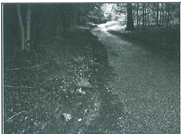
Erosion route du Câtelier
